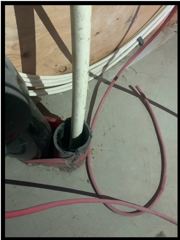
Figure 6: Cutouts and Poor Seals Create Gaps in the Foundation. (a) Remaining cutout left unfinished after occupancy (top left). (b) Gravel visible around sump (top right). (c) Gaps remaining around electrical conduit (bottom left). (d) Plumbing Cut-outs Remain Unsealed near bathtub (bottom right). All photos Chantal Wilson, from site visits for this study.
