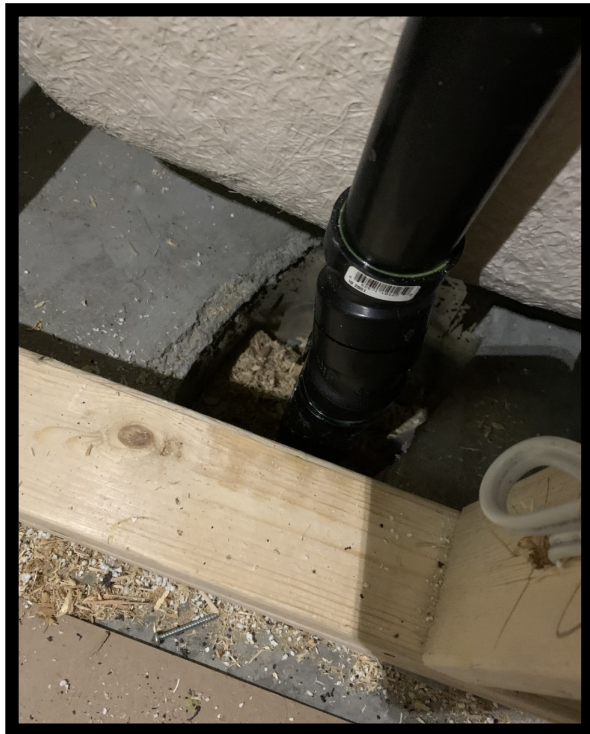
Figure 6: Cutouts and Poor Seals Create Gaps in the Foundation. (a) Remaining cutout left unfinished after occupancy (top left). (b) Gravel visible around sump (top right). (c) Gaps remaining around electrical conduit (bottom left). (d) Plumbing Cut-outs Remain Unsealed near bathtub (bottom right). All photos Chantal Wilson, from site visits for this study.
