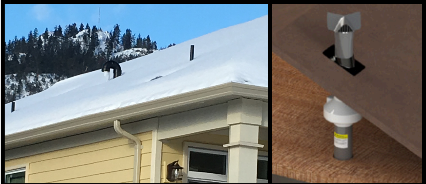
Figure 12: Terminations. (a) Left: Frozen J Hook Termination on Vent Pipe. Photo Courtesy of John Kostelnick, Okanagan Radon. Not taken for this study.(b) Right: Specially designed radon vent pipe termination. Ipex Inc. RadonX Product Brochure
